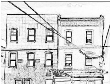
example of mis-aligned and mis-matched roof cornices
